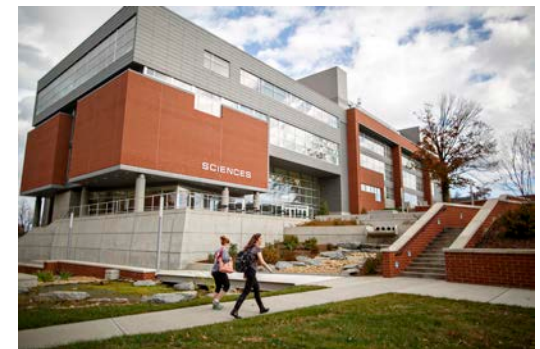
New Science Building, Constructed 2014-2016
