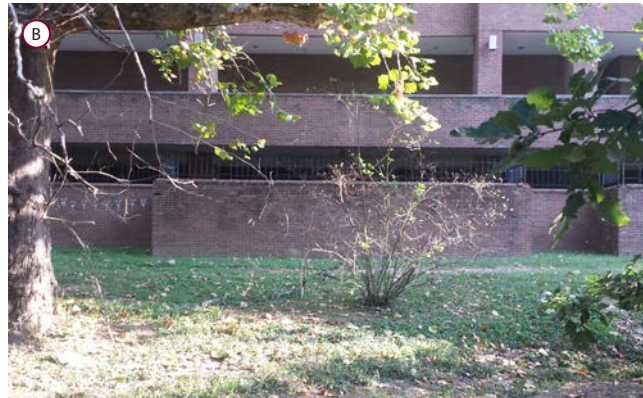
South Elevation of Campbell Building
