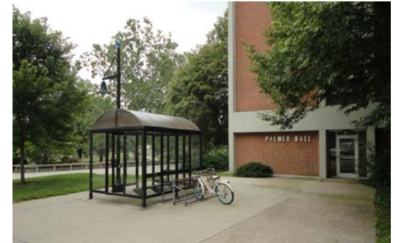
Existing Bus Shelter
