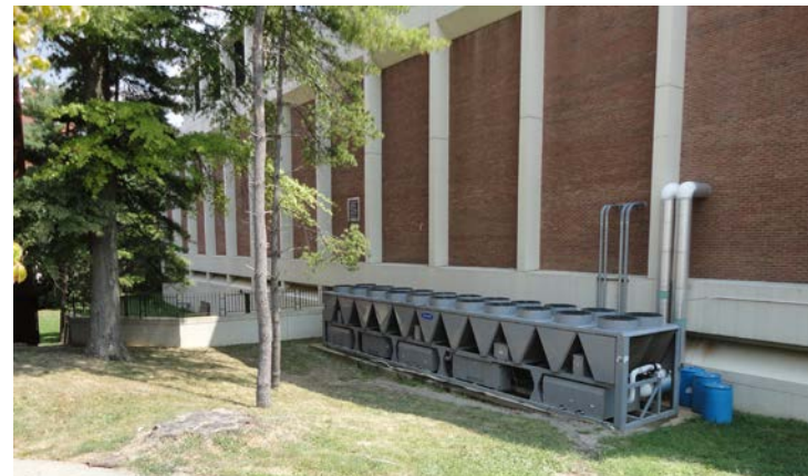
West Side of Powell Building
