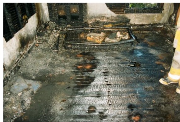
Fig. 7 Scene photograph of suspected ignitable liquid pour (Wood et al. 2012)
